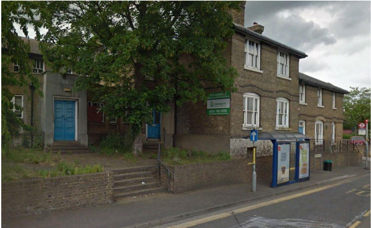
Photo 3. View of site (looking NW)
